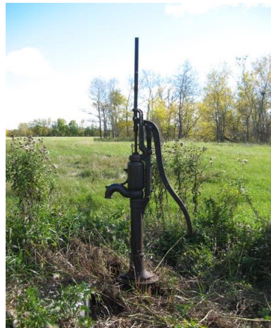
An old-fashioned hand-pump and well located south of Fraserwood, prior to sealing by the EICD.
