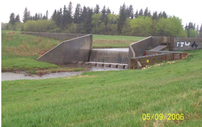
Photo 10. Gradient control structure and modified Denil fish ladder (on right).
