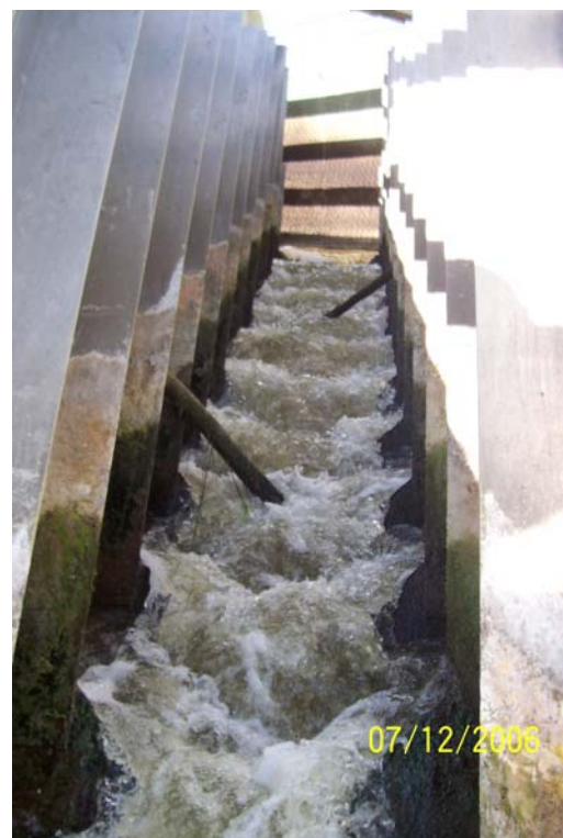
Photo 11. Flow conditions observed at the downstream side of the gradient control structure fish ladder, July 12, 2006.
