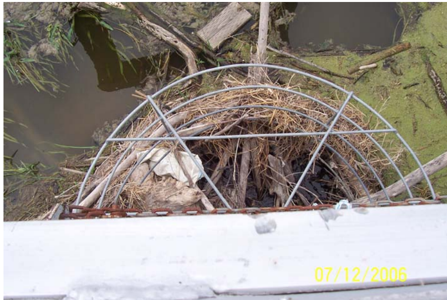
Photo 12. Debris clogging upstream end of fish ladder.
